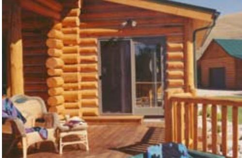
The unique characteristics of wood make it suitable for a variety of applications in the building industry: log or timber homes, decks, rough-sawn siding, fences, and shingles. Without protection from sun and moisture, wood "weathers" and deteriorates. Finishes are used to enhance appearance and dimensional stability, and to prevent deterioration.
